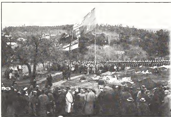
Fig. 10. Laying the foundation stone of the Albany Museum (1897).
